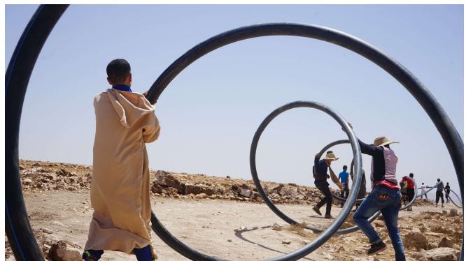
Figure 4: Community members uncoiling HDPE pipe
