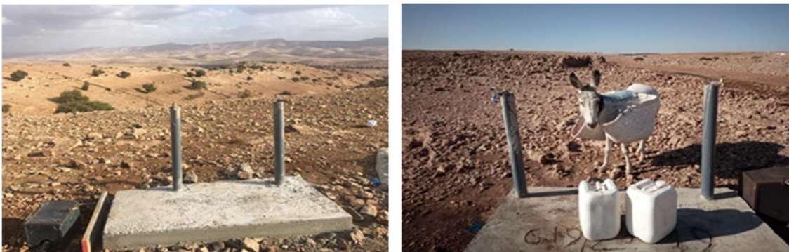
Figure 6: Completed domestic (left) and livestock (right) tapstands
